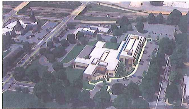
An aerial view of the expansive, integrated health facility.
