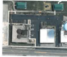
Walkertown Town Hall with parking located to the side and rear of the building
