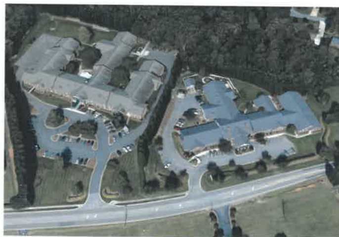
Robinwood Senior Living apartments located next to Kerner Ridge Assisted Living facility in Kernersville.
